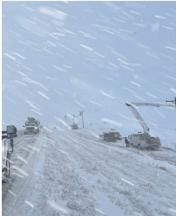
Line crews work to restore power along highway during winter storm.
