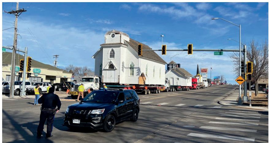
Two buildings are moved from Augustana University campus due to expansion of the college athletics complexes.
