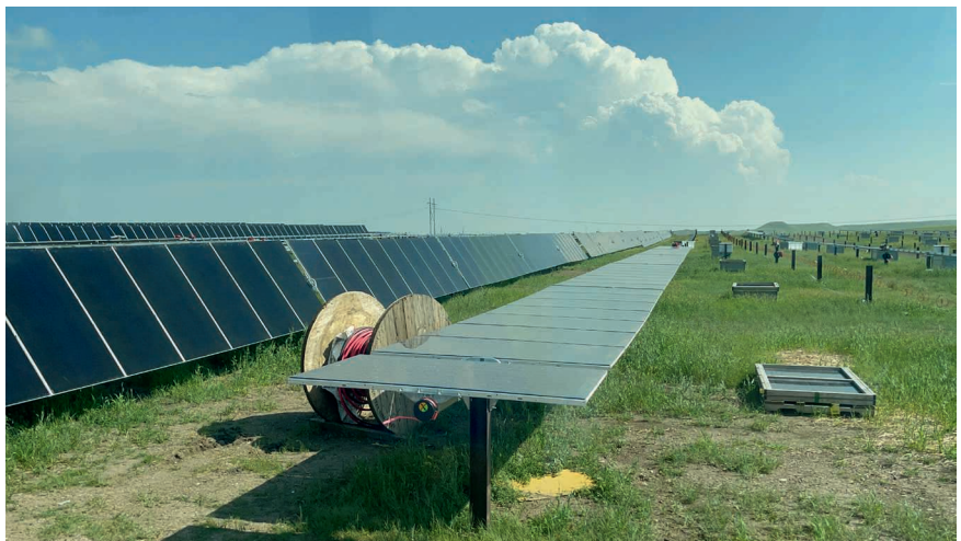
A look on the ground as crews prepare the Wild Springs Solar Project for power generation. Photo submitted by East River Electric
