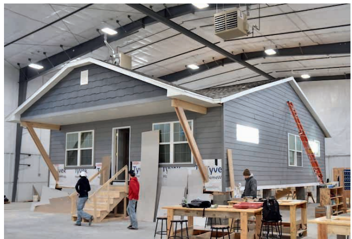
Students in the Harrisburg School District's home builders academy have built a full house. Photo courtesy of John Klemme
